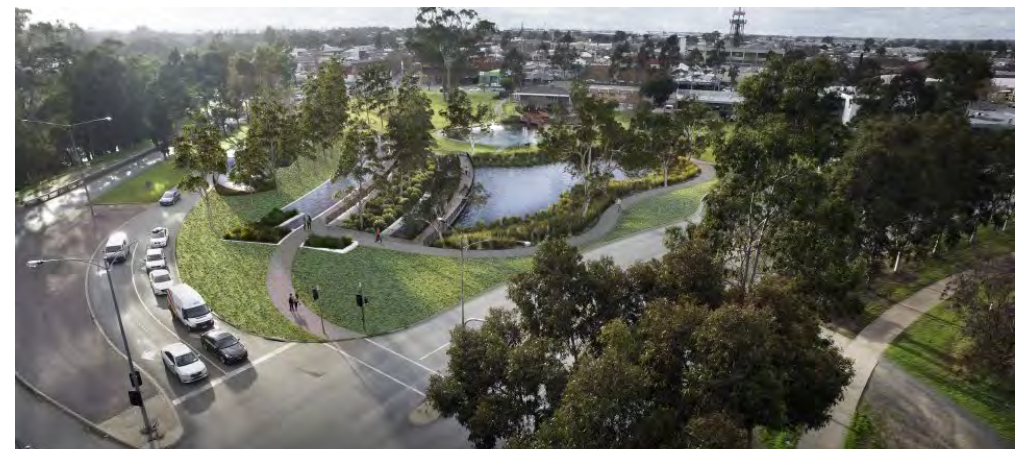
Lake Stormwater Harvesting Scheme, Shepparton Victoria
