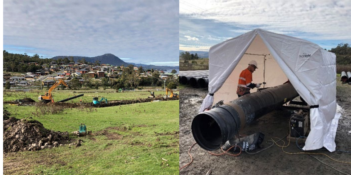
Fenton Line Trunk Water Main Upgrade
